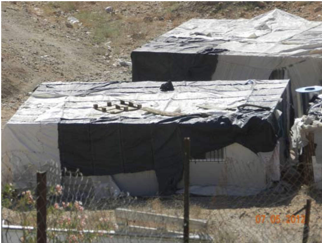
Prefab buildings brought in without permits by Bedouin in the Mishor Adumim area, next to Route 1.
