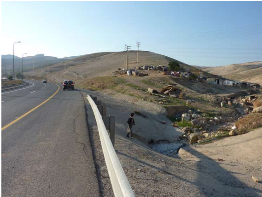
Illegal building by Bedouin next to Route 1.
