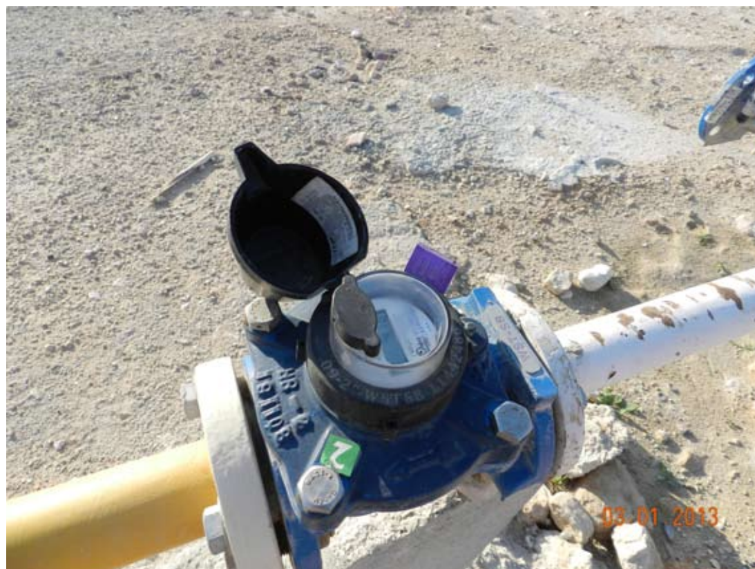
A water meter installed by Mekorot, Israel's national water company, next to an illegal Bedouin construction site near Nahal Og.
