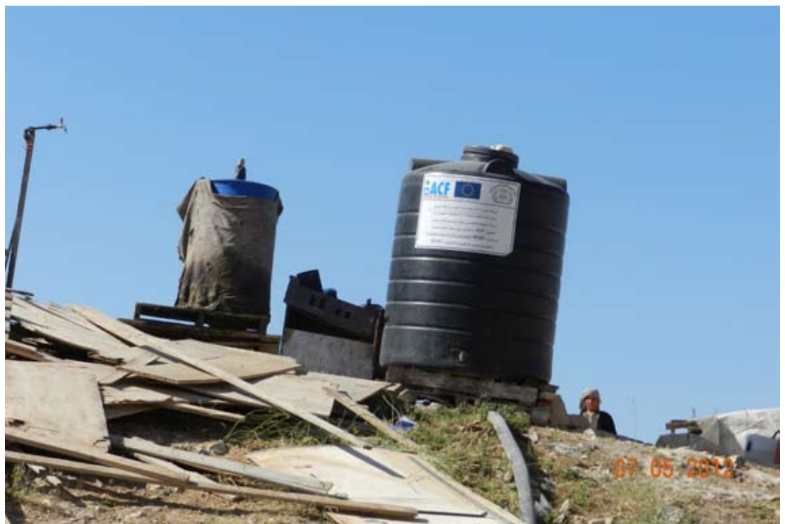
Water tanks at an illegal construction site in the Maale Adumim area, supplied by the humanitarian organization ACF and the European Union.
